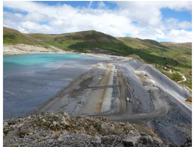
Figure 3. Mine tailings are often stored in large impoundment ponds. The EOR is an important part of the team that monitors the stability of the tailings storage facility.
